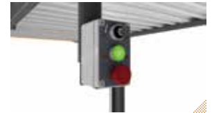
Key switch for each operation with emergency stop button
